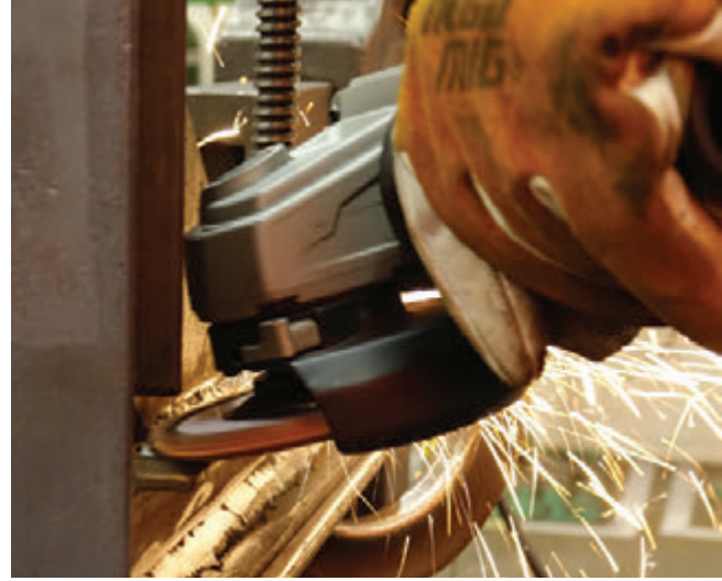
Blending fillet welds to ensure proper penetration prior to inspection.
