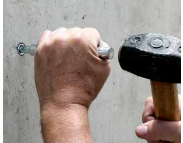
Anchor being set with hand tool.
