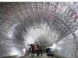
Tunnel insulation
