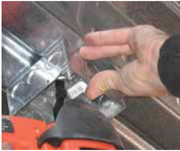
MP034TH fastener used to attach a junction box
