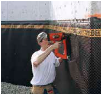
Waterproofing to concrete
