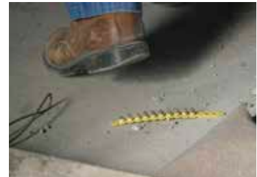
No more fines for unspent loads on the jobsite.
