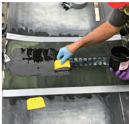
Before Metal Clips Splice Repair
